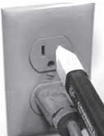
AC Voltage in wall receptacles
